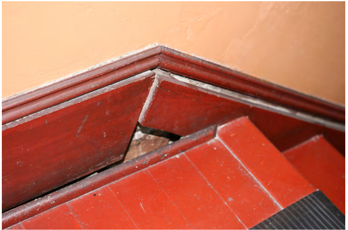
CP 47. Southwest Stair, Panama Ho- tel showing separation between the stair and the masonry wall
