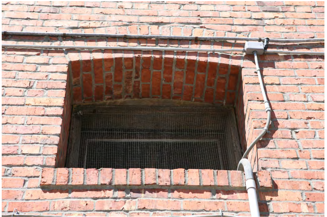
CP 5. East facade, Panama Hotel, showing arched window opening with an added screen and electrical conduit
