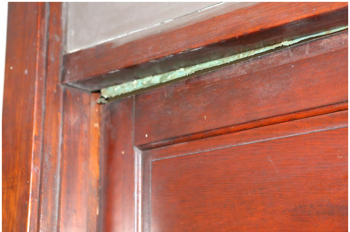
CP 42. Corridor, 4th Floor, Panama Hotel showing offset between a door and its frame
