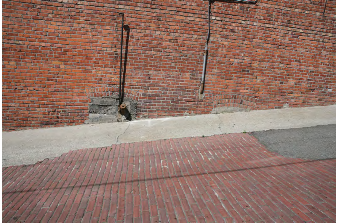
CP 3. East facade, Panama Hotel, showing in-filled window open- ings and miscellaneous pipes
