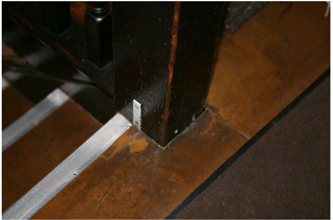
CP 43. Main Stair, Panama Hotel showing temporary connection reinforcement at the newel
