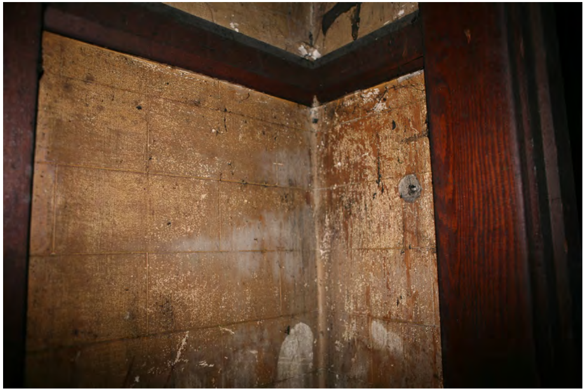
CP 17. Detail of scored walls, basement corridor and bathroom
