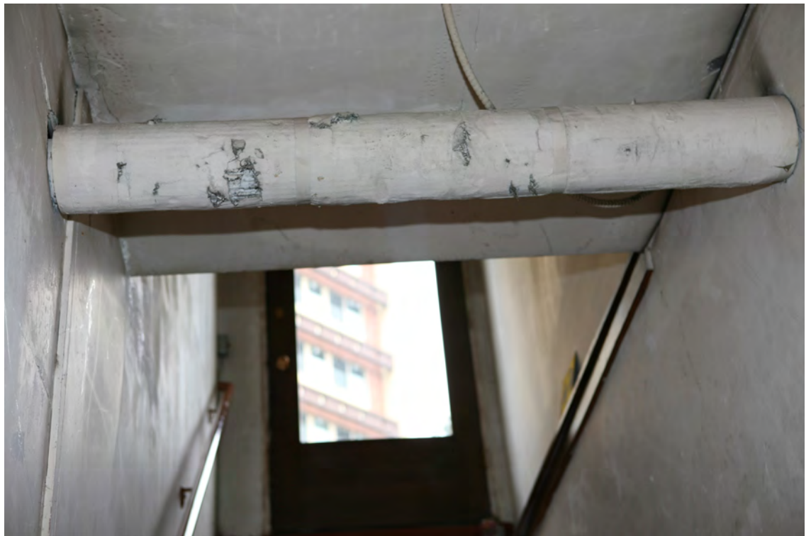
CP 46. Northeast stair showing wrapped pipes running over the stairwell
