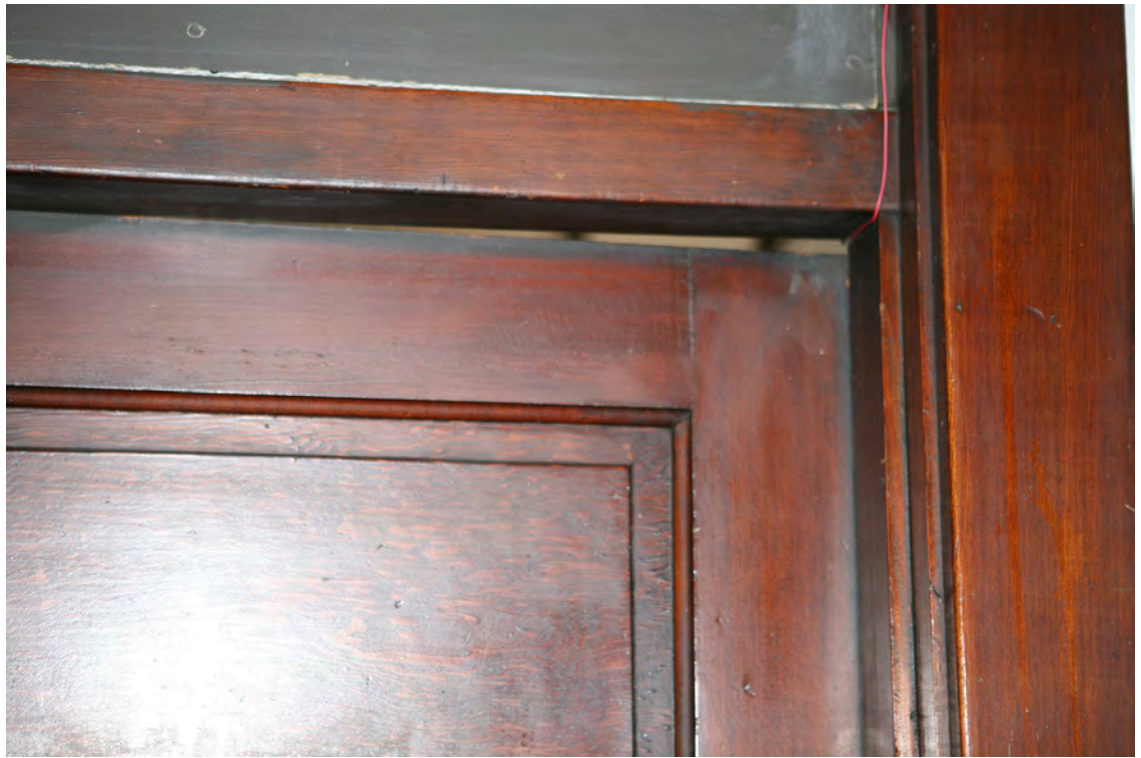
CP 41. Corridor, 4th Floor, Panama Hotel showing the offset between doors and their frames due to settlement along the south wall
