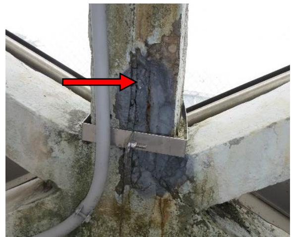
Figure 17. Removed spall within the body of the precast element. Note missing grout between precast members.
