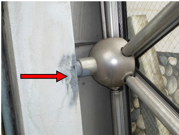
Figure 14. Removed spall at connection location. Note: connection is painted with blue colored coating.
